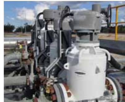
6 x 200 mm, 100bar ash lines, Electric Actuation
