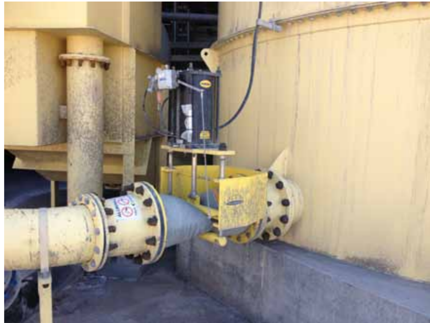
Tank level control valve - smooth flow deflection
